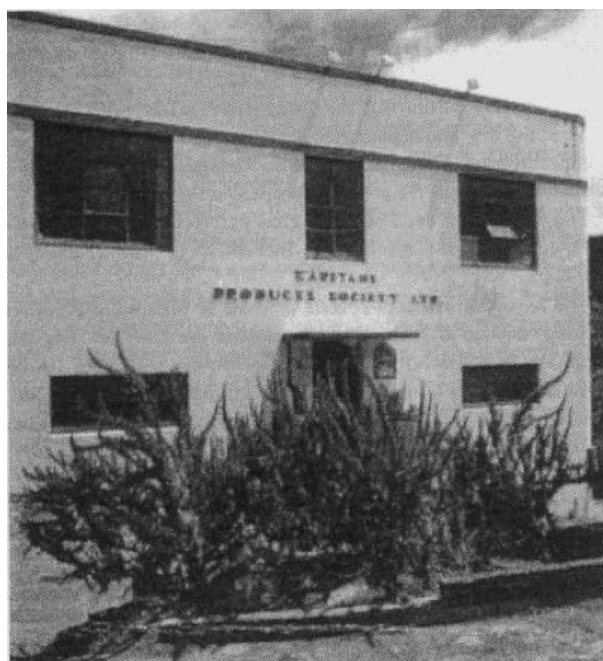
Fig. 3. The Karitane Products Factory in Melrose, Wellington, where during her employment as a laboratory assistant, Shorland's biographer probably first encountered Brian Shorland. The building, designed by prominent Wellington architect William Gray Young, is near the Karitane Hospital and Sir Truby King's residence. It has a category 1 rating on the NZ Heritage List and is currently used as residential accommodation. [Photo: http://nzetc.victoria.ac.nz/tm/scholarly/ChaStra-fig-ChaStra230a.html ]. For modern views of the building and its environs, see: http://www.heritage.org.nz/the-list/details/4431 .
