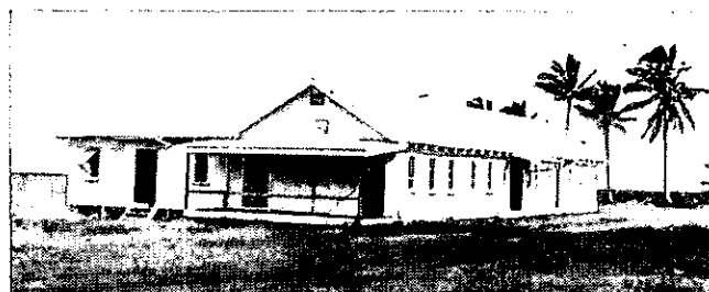
The new School of Education building.
