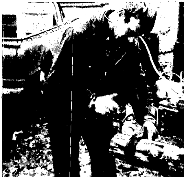
Step 1. The fitting of three rings over the end of the log. The first ring (steel) is secured with some six steel wedges to prevent its movement towards the end of the log. The next ring which has a w contour on its outer surface is made of rubber. The third ring is of steel and free to slide.
