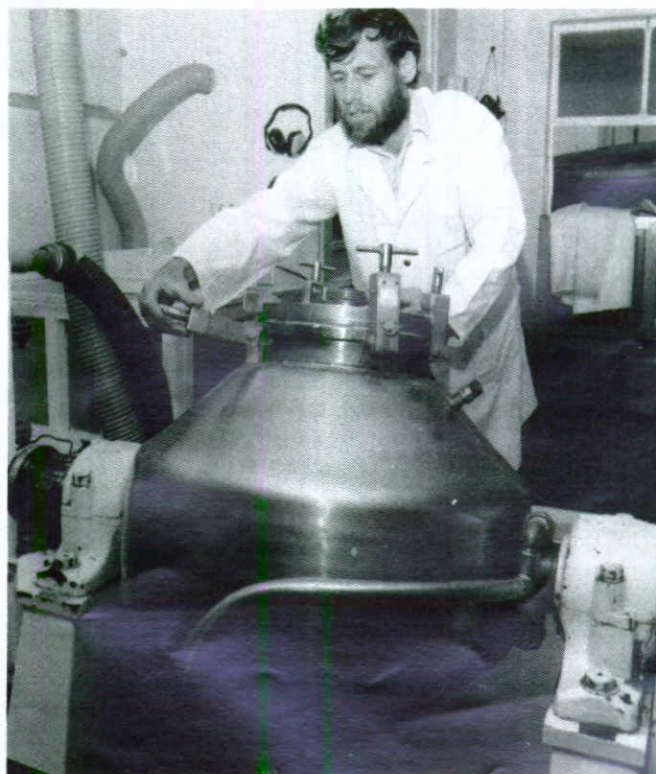
Figure 8 The rotating pressure vessel at the Biochemical Processing Centre (DSIR, P.N.) used to prepare the first batches of high capacity SP cellulose.
