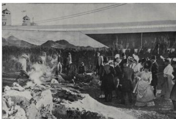
Fig. 1. Early promotion of a geothermal area as a tourist attraction: 'Geyserland' at the 1906-1907 exhibition in Christchurch.
