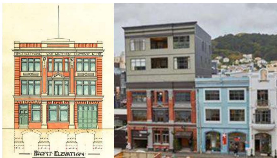
Fig. 2. Warehouse and offices of NZ Acetylene Lighting Co., 5 Tory Street, Wellington, 1917. Architect: Crichton & McKay. The floor plans indicate a show room, office and store on the ground floor with an internal lift connecting the store to two upper floors. The use of the upper floors is not indicated on the drawings. The parapet was removed in 1936, as a response to the 1931 Hawkes Bay earthquake. (Image: Bulleymont Fortune Architects Archive, used with permission). An architecturally unsympathetic two-storey addition made to the building around 2000 attracted the comment "they have reinvented cool", when the building was recently for sale.
