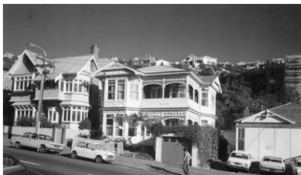
Fig. 2 (continued). Looking east from Victoria University to former residences on the west side of Kelburn Parade in 1976, prior to their removal or demolition for the construction of the Murphy building. No. 30 is at the extreme right of the photograph. By the mid-1970s, the front of the building had been substantially modified and its front garden and picket fence replaced by a car-park (Image by Charles Fearnley, Wellington City Recollect, Reference 50003-2309).
